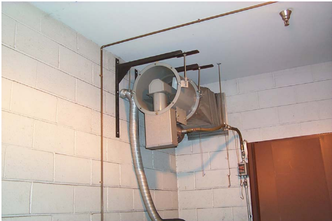
Flammable Storage/Mixing Room: Exhaust system (note sprinkler head)
