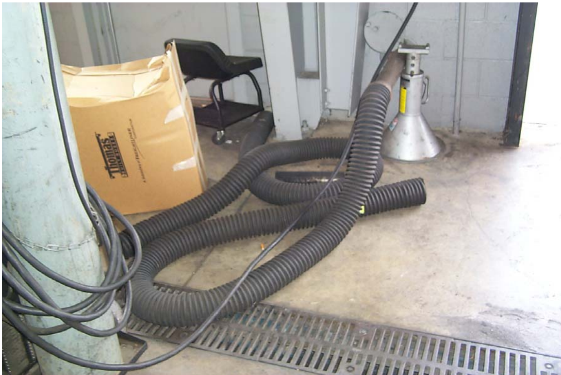
Maintenance Bays: Engine emissions exhaust port and trench drain
