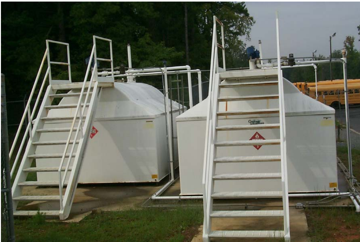
Above-Ground Fuel Storage Tanks
