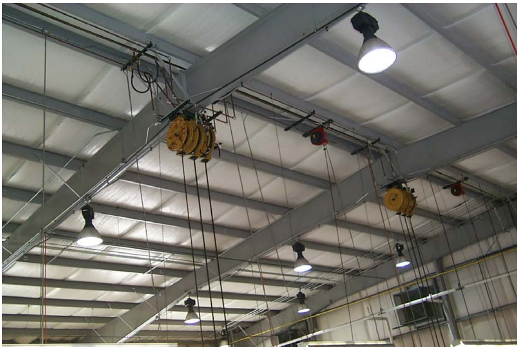
Maintenance Bays: Overhead reels
