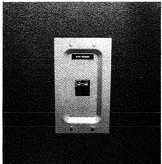
Figure 4-6. Over-Current Circuit Breakers
