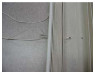
Fig. 3 Starting at top rail, thread string through holes as illustrated on diagram
