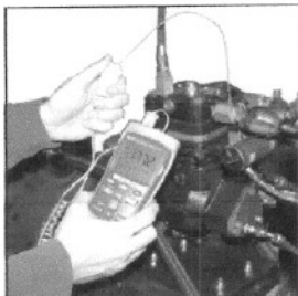
Testing the temperature at the discharge fitting.
